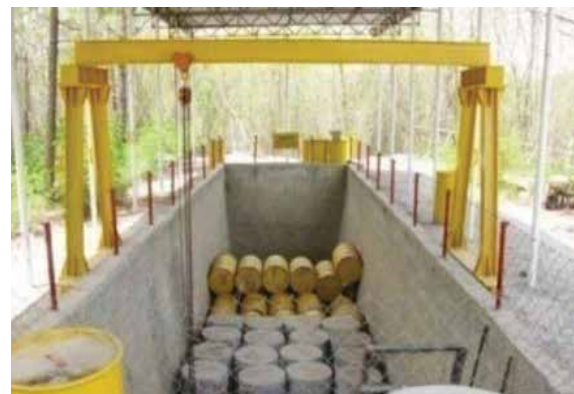
PINSTECH Predisposal Radioactive Waste Management Facility (PPRWMF)
